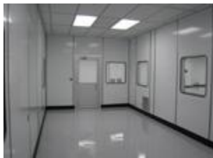
Custom Designed Clean room
